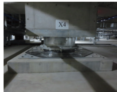
Gotenyama SH Building
